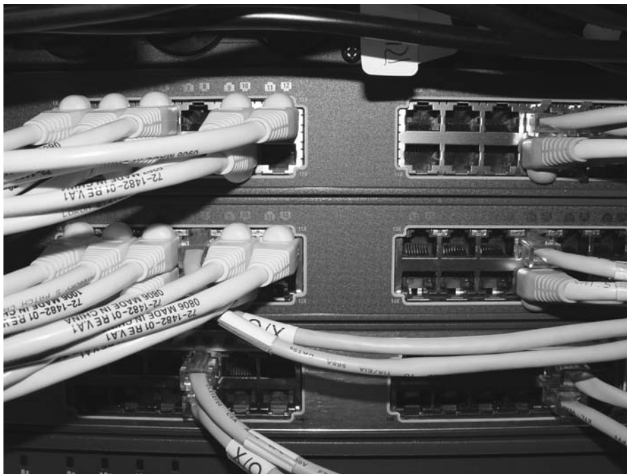
FIGURE 20.3 Rack-mounted switches
